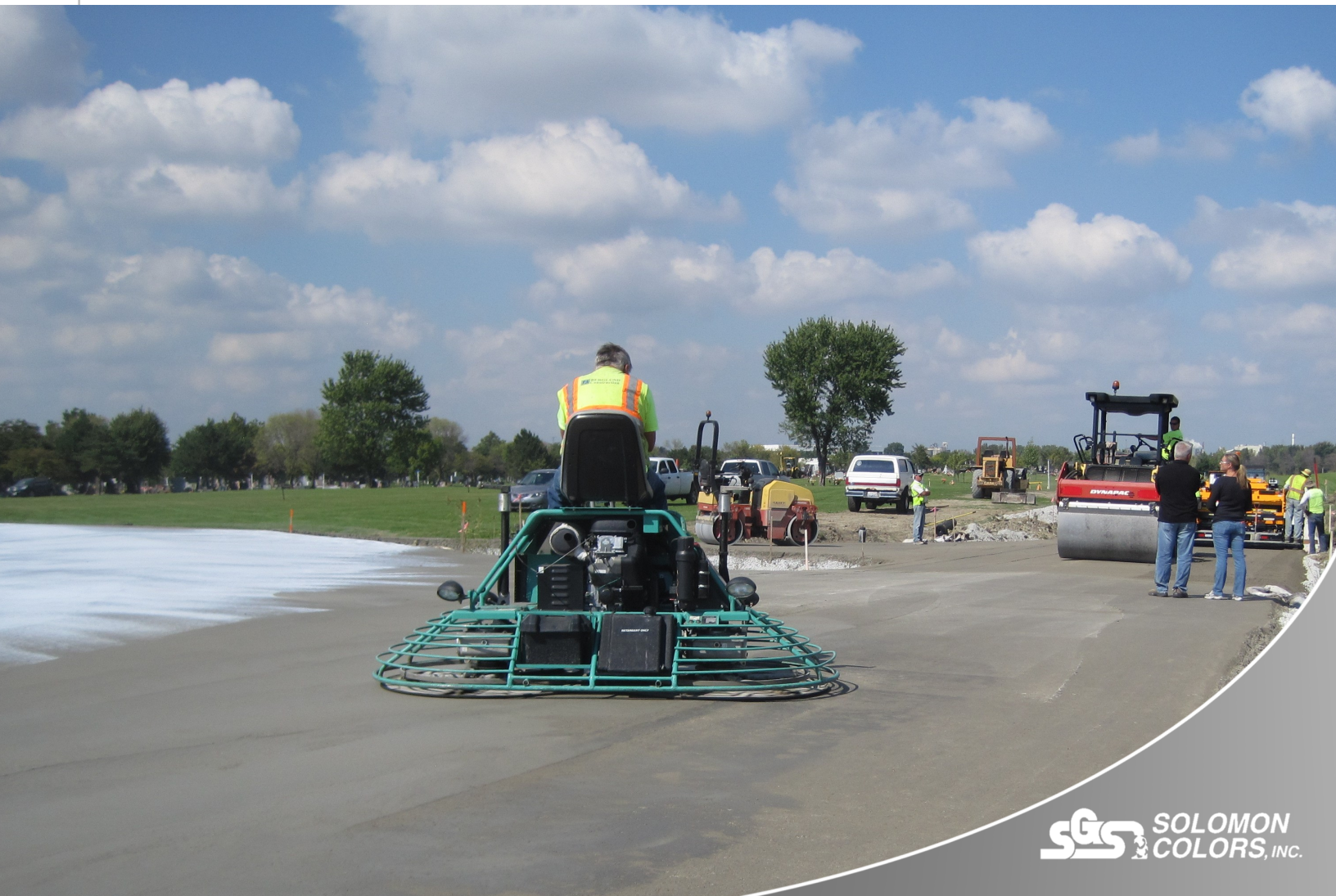
RCC Broom Finish
