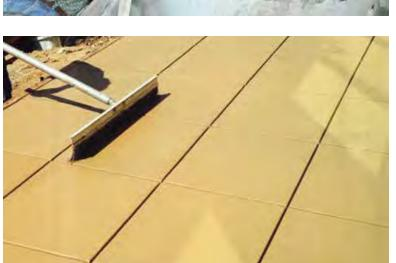
DRY 1-25 LB. BAG PER 4 YARDS/6.25 LBS. OR COLORFLO 1% LOADING Produces soft colors, performs best when stamping with one (or more) darker Antique Release. Accent this loading with Color Hardeners or stains to produce, natural, multiple colors. If a broom finish is desired, keep concrete at a 4" slump, and use a damp — but not wet — broom.
