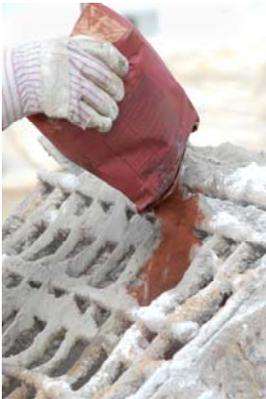
Synthetic and Natural Iron Oxide Pigments have historically been the primary color used in concrete masonry. In addition, Chromium Oxide is used to produce shades of Green. Cobalt Blue is used for the blue shades. Iron Oxide's, Chromium Oxide, and Cobalt Blue are permanent, inert, stable to atmospheric conditions, and sunfast. They all comply with standards set by ASTM C979 "Pigments for Integrally Colored Concrete".
