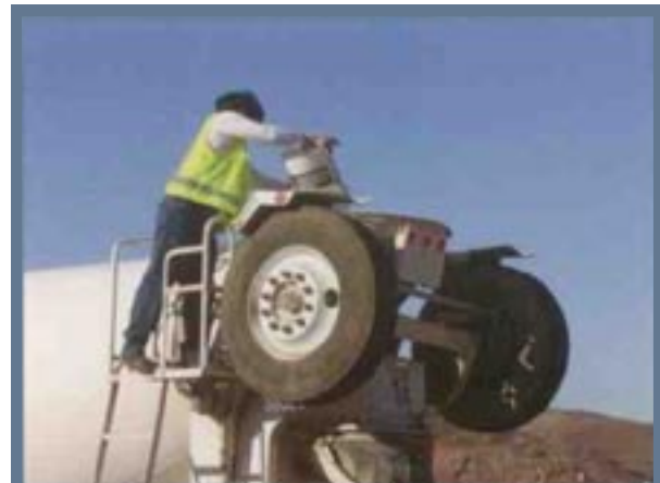
Adding Fibers to the Truck
